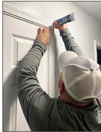
Kirt Wilson sealing around a door in a recent job
